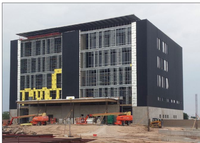
Construction on the new Lea County Judicial Complex in Lovington, which is scheduled to open in June 2019.
